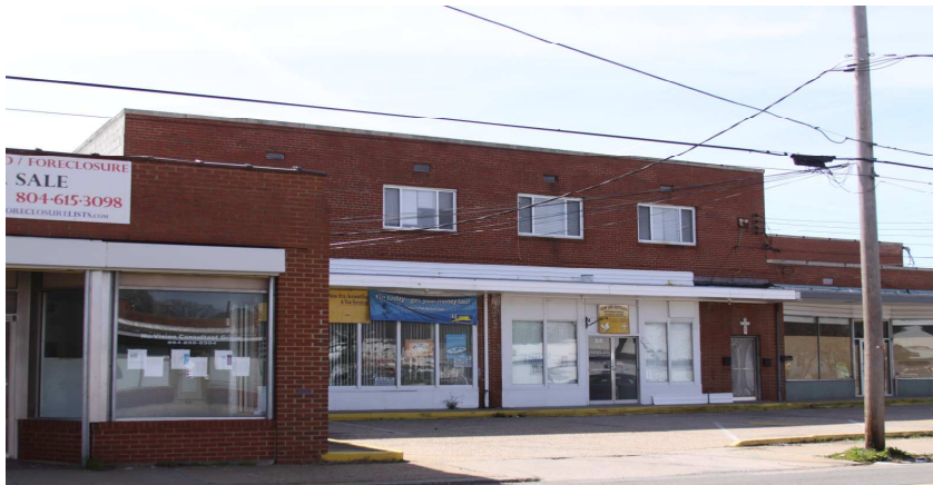
Buildings like this one, located in Richmond's Fulton neighborhood's commercial corridor, are great places for small businesses to renovate and improve. LISC hopes the loan will stimulate the economy in city neighborhoods like this one.
